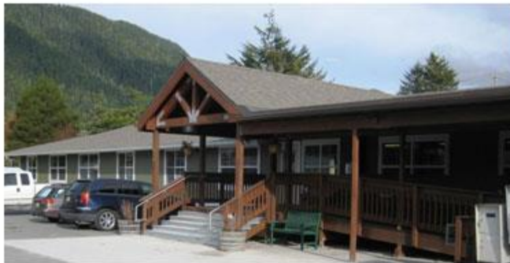
New roof and covered entries at all buildings
