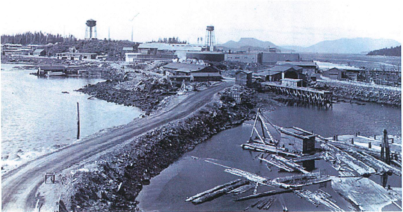
Historical view of the Japonski Island Boathouse (right of center) during World War II. View is from the top of a gravel conveyer. The causeway in the foreground is adjacent to the current bridge across the channel. Photo Sitka Historical Society, Johnson Collection.
