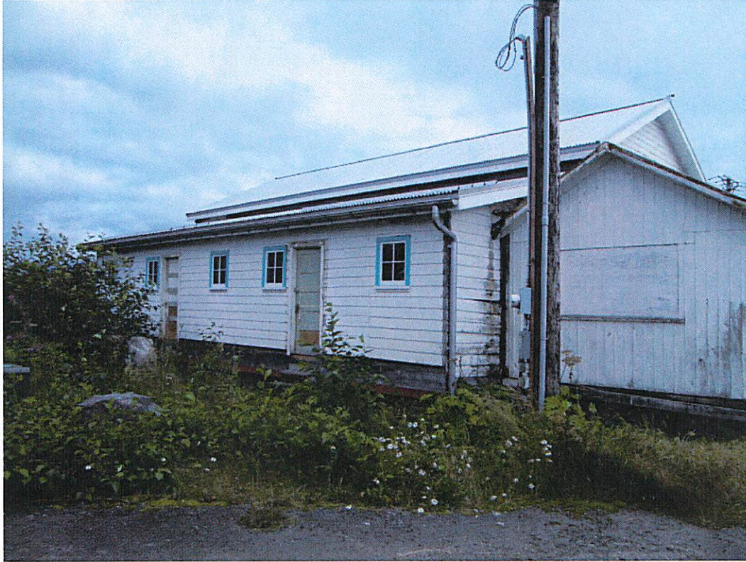
Above, north side (before removal of addition). 7/30/16.
