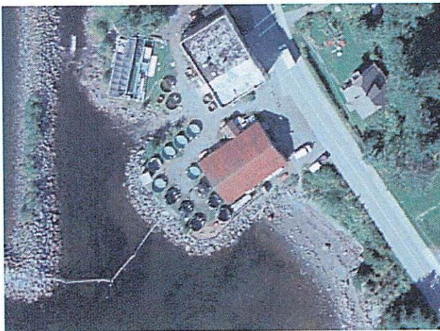
Left: Contemporary satellite imagery showing the present-day site, showing the Mill building's axis relationship to Lincoln Street.
