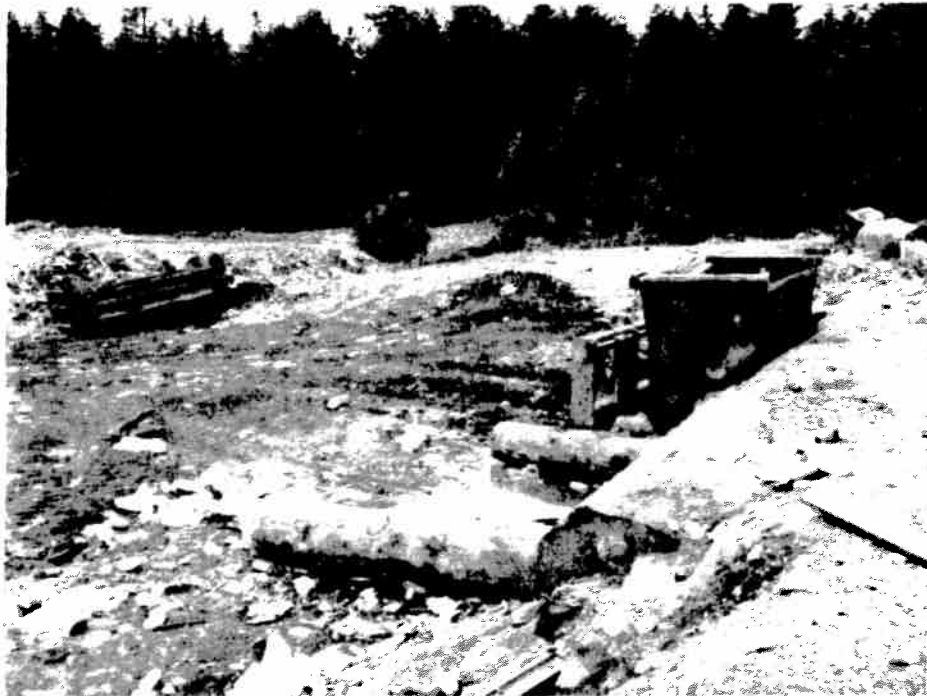
Public Dumpsite (Standing Water and Excessive Litter)
