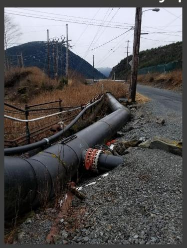
Pumped supply ties into 42" Raw Water line. Other concerns with pumped supply is not available when Blue Lake turbines offline, power out and potential saltwater intrusion on higher tides.
