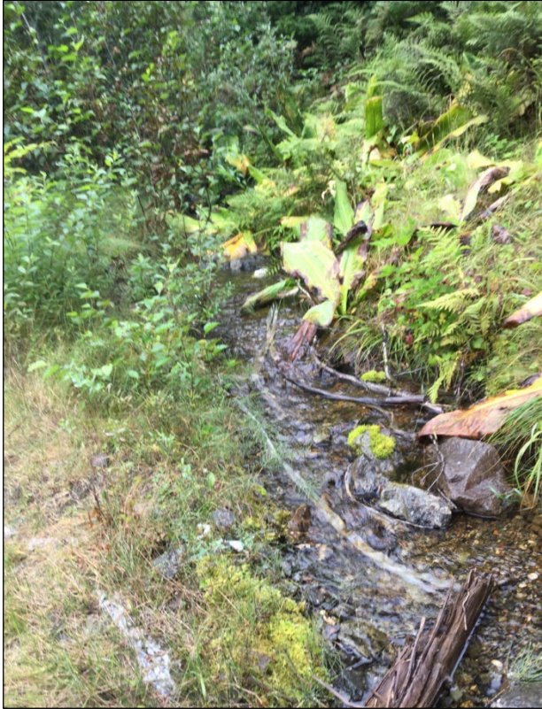
Figure 1.–Drainage upstream and adjacent to Comet Beach Road.
